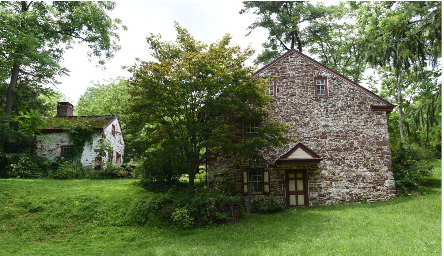
Daniel Boone Homestead – Exeter Township
